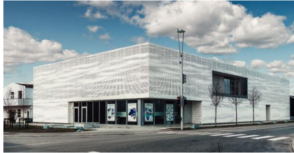
Figure 14: Machine room at Århus Ø where the heat pumps are located [Kollision, 2020].
