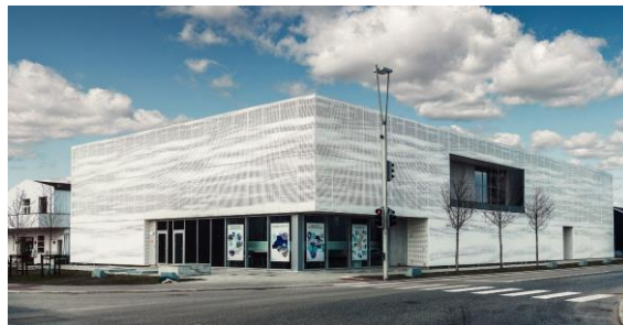
Figure 2: Build at Århus Ø where the heat pumps are located [Kollision, 2020].
